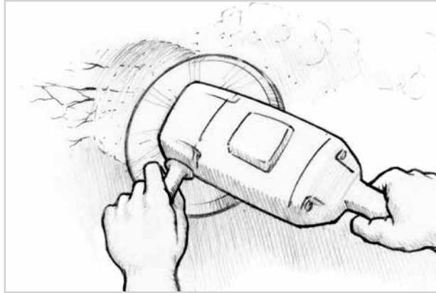
Figure 2-3 Grind out an area of many closely spaced or deep cracks with a disk grinder.
